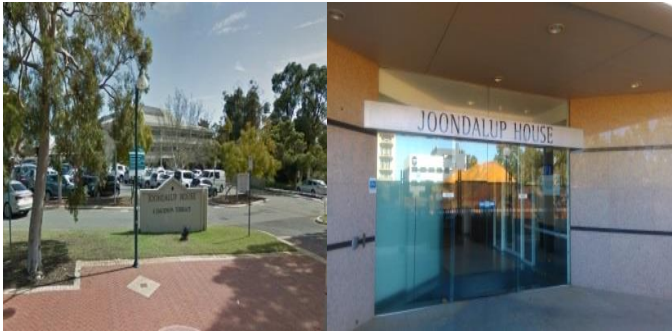
Joondalup House, 8 Davidson Terrace Rear Building
